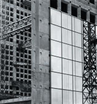
Placing of the facade and supports between the two pylons, June 1987.
