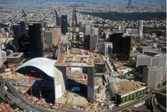
The Grande Arche under construction, 1985-1989, the building of the flanks and the placing of the roof .
